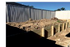
**Timber Sleeper Retaining Walls**
