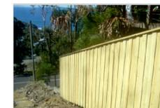
**Double Lap & Cap Treated Pine Timber Fencing**
